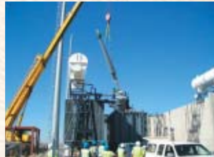
● Mounting 800kV bushing
