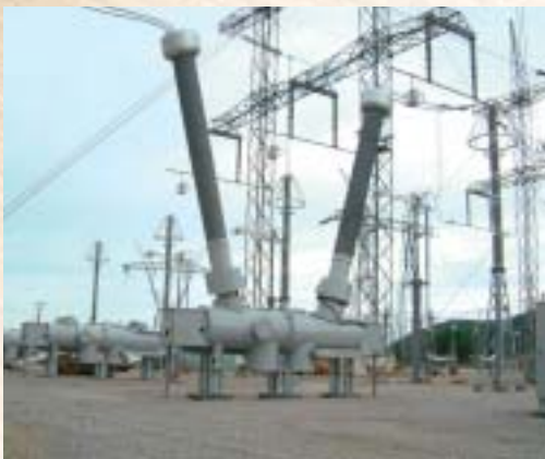
● Installation of GCB at substation
