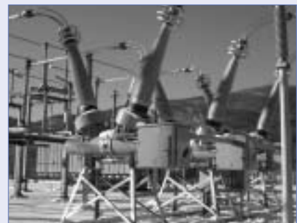
362kV dead tank type gas circuit breaker
