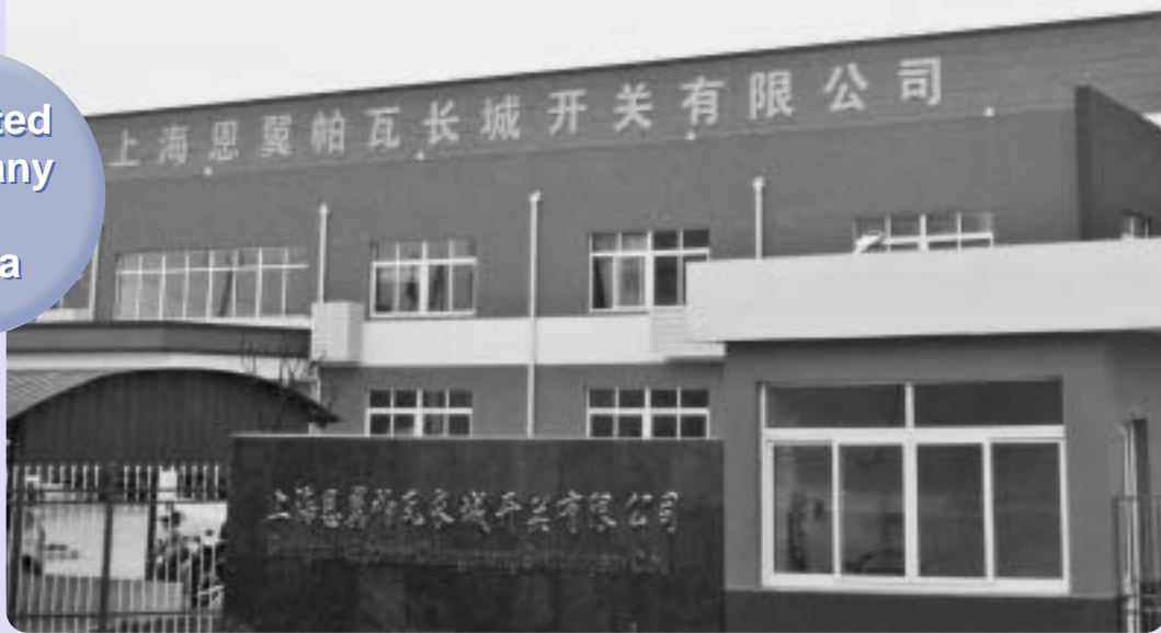
New plant inaugurated in August 2010
