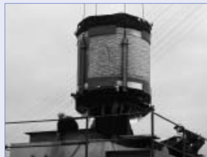
Hoisting the winding of an aged transformer
