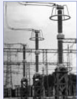
266kV polymer insulator type lightning arrester
