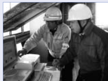
Checking the combustion status of the boiler
