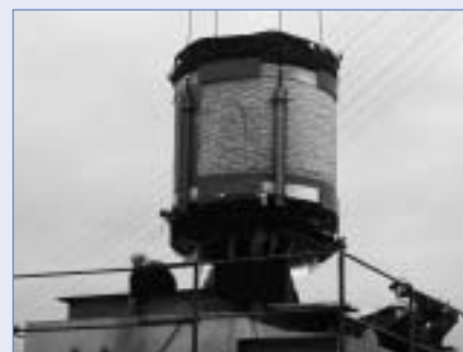
Hoisting the winding of an aged transformer
