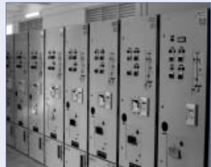
24kV dry air-insulated C-GIS
