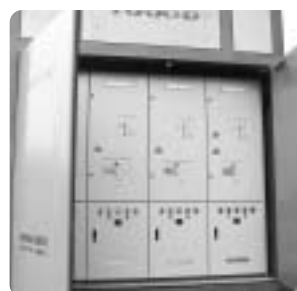
40.5kV C-GIS for Qinghai line
